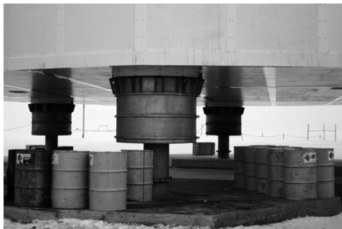
Pilotis hydrauliques Station CONCORDIA
